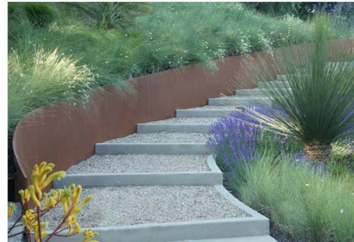
INDICATIVE PATHWAY/STEPS AND SMALL RETAINING SYSTEMS PROPOSED INCLUDING CORTEN STEEL AND SMALL STONE ON DECOMPOSED COMPACTED GRANITE.
