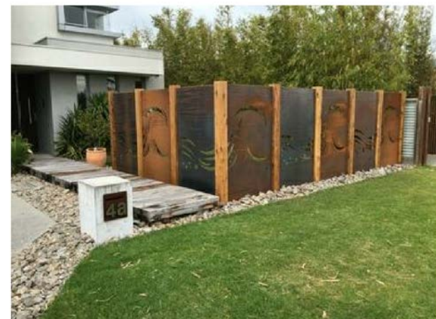
INDICATIVE RESIDENT PRIVACY SCREEN SYSTEMS PROPOSED INCLUDING LASER-CUT CORTEN STEEL AND HARDWOOD.
