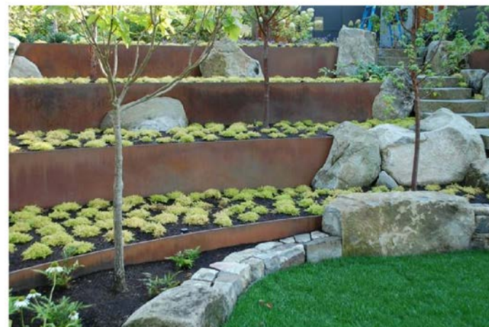
INDICATIVE TERRACED RETAINING SYSTEMS PROPOSED INCLUDING CORTEN STEEL AND LARGE STONE.
