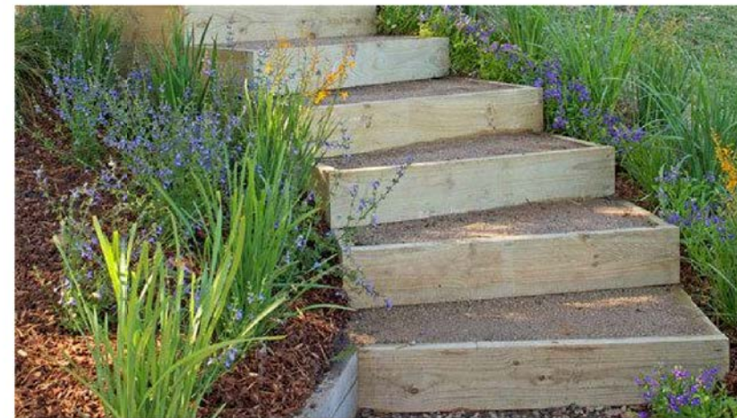
INDICATIVE STAIR SYSTEM PROPOSED IN APZ USING FIRE-RESISTANT TIMBER SLEEPERS.
