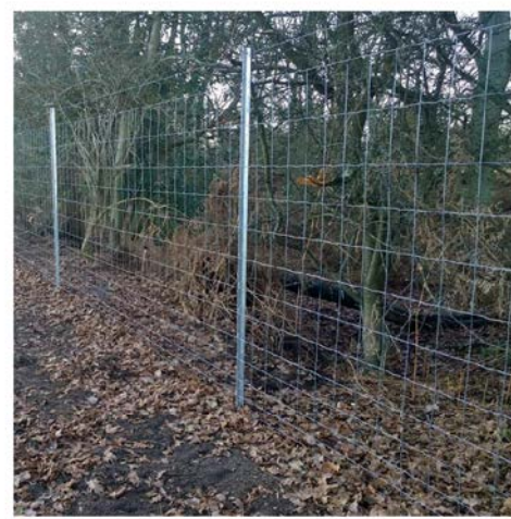
TYPICAL DEER EXCLUSION FENCING DETAIL PROPOSED INCLUDING RINGLOCK MESH 2100 HIGH AND GALVANNEAL STEEL POSTS AND STRAINERS.
