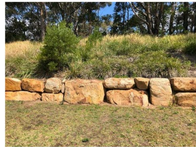
INDICATIVE MEDIUM RETAINING SYSTEMS PROPOSED INCLUDING SANDSTONE GRAVITY BLOCKS.
